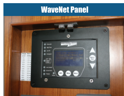
Typical WaveNet junction box installation. (Part number 22-92610 installed on M773LW3, shown with optional sound enclosure)
